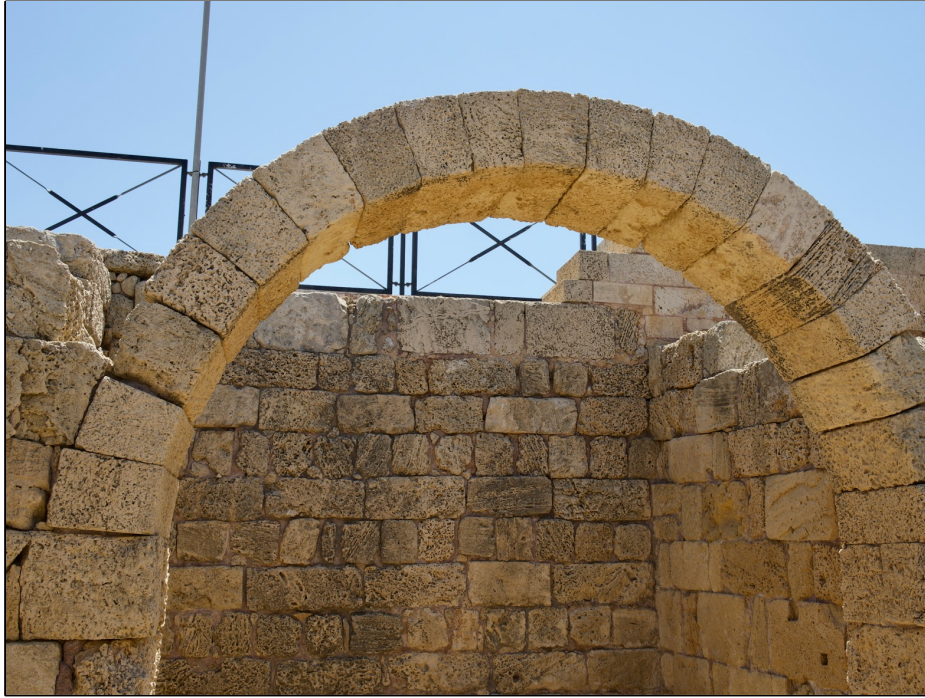
Example of a Roman Arch. With this type of arch, the center keystone is larger on the top than the bottom, which allows all subsequent stones to form the arch.
